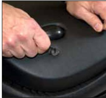
2. Using a 5/32" Allen wrench, remove the screws securing the outer shell to be replaced from the
